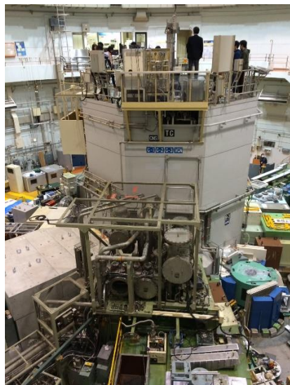
Photo A. Kyoto University Research Reactor.
