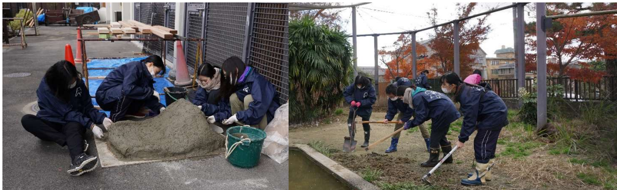
Fig. 1. Left: The making of the artificial rock for the penguins; putting sand and cement mixture onto the wired mesh. Right: Ploughing the ground for the flamingo house.
